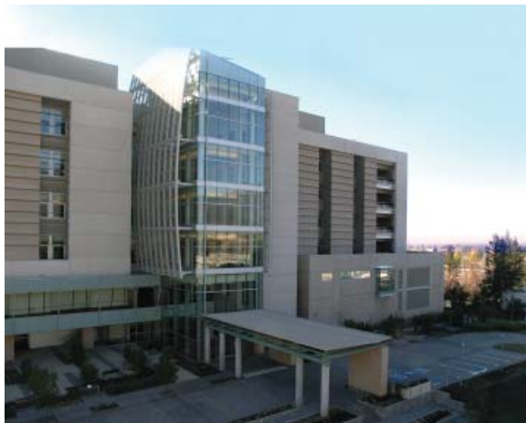
City of Hope National Medical Center in Duarte, California.
